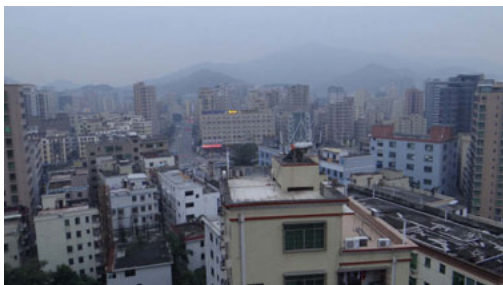
Fig. 8: Typical aerial and eye level image of urban structures outside the former SEZ
