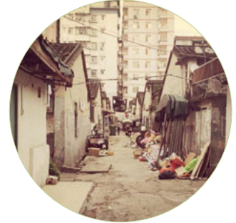
Figure 8.1.2.3 The main path in tangtou housing are abandon and full with trash
