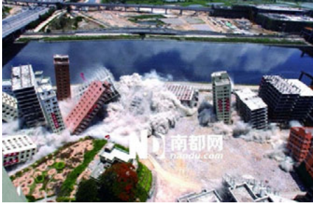
Figure 2.2.5.2 The blasting of Yunong village in Futian District, known as " China's first demo ", is the epitome of transformation of urban village in Shenzhen Source: http://paper.oeeee.com/nis/201308/09/93568.html
