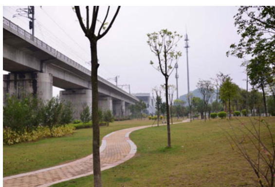
Figure 29. Public space in lack of use and maintainance
