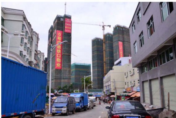
Figure 20. New commercial real estate projects in old town
