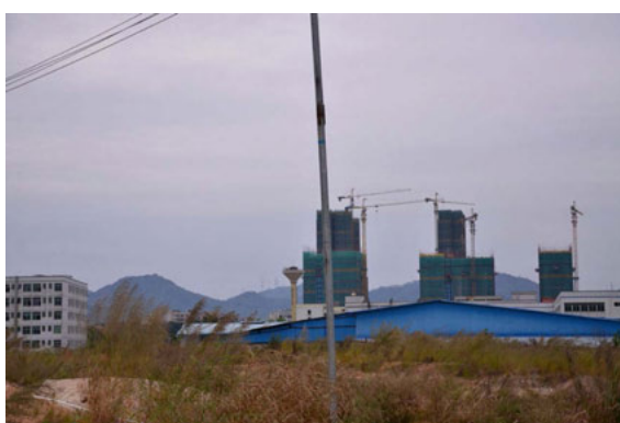
Figure 27. A lot of projects are still under construction
