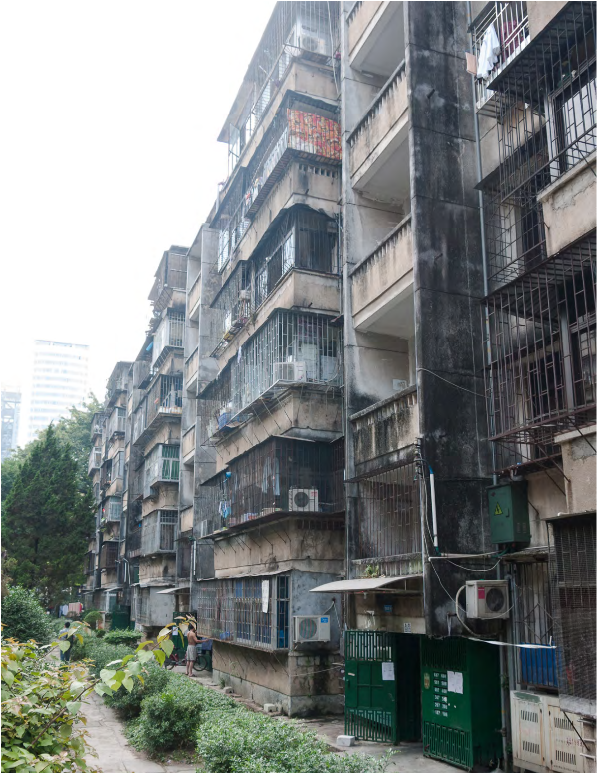
Residential building (Photo by author)
