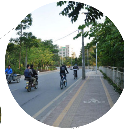
Fig 2.3.6 Existing greenway in a good quality
