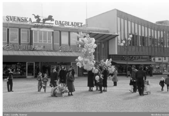
Historical image of Vällingby Centrum in the 1950s
