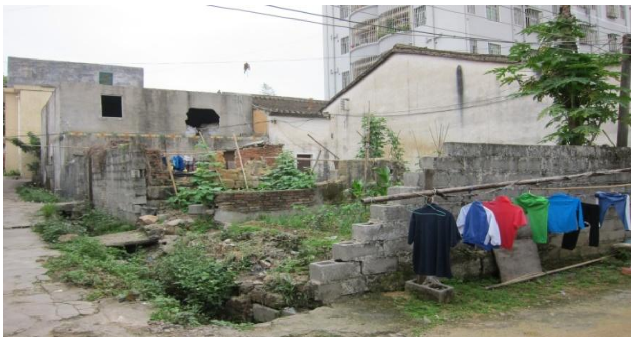
Figure 47: street scene "extension" zone
