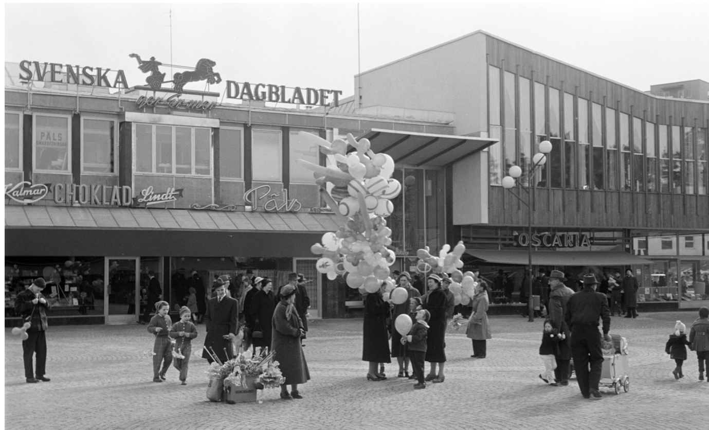
Historical image of Vällingby Centrum in the 1950s
