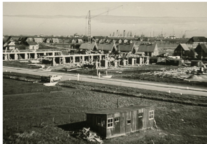
Plan West, construction works for the new Zeeheldenbuurt (1957) Source: municipality of Nissewaard
