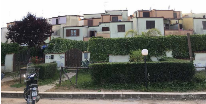
The Indians' apartments (top) and the larger villas owned by Italians (bottom) strike a surprising contrast, yet are part of the same neighbourhood.
