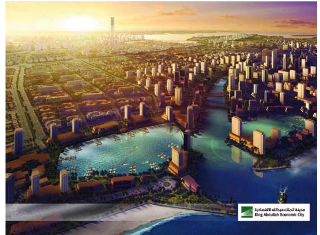
Looking east from the Phase 1 Bay la Sun and Esmeralda developments, one of the canals leads back to the eastern edge of KAEC.
