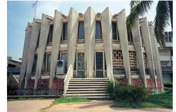
The Phnom Penh Teacher Training College designed by Vann Molyvann, completed in 1972.
