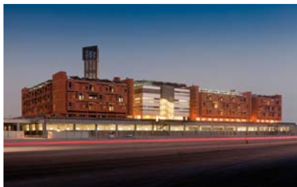
The MIST campus is part of the first construction phase. The roof is covered with solar panels and a low-tech wind tower. The simple construction uses age-old convection technology to pull cooling breezes into the courtyard.
