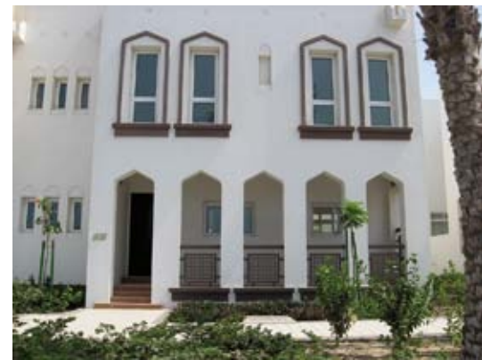
Houses under construction in The Wave ITC development, southeast of The Blue City. The white, flat-roofed architecture is consistent with planning regulations, 2010.
