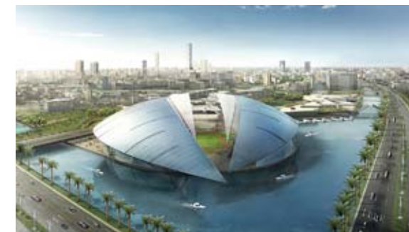
Designed by SOM, Rabigh International Stadium at the edge of the CBD juts into the dividing waterway.
