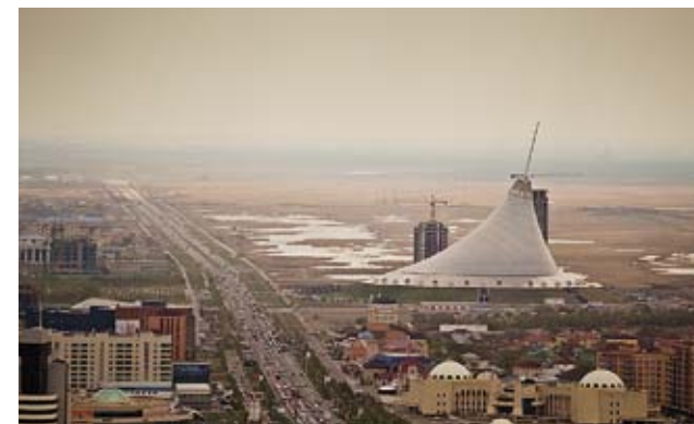
The Khan Shatyr is a 150 m high tent structure designed by Foster + Partners in 2006. The transparent 'skin' covers 140,000 m 2 of shopping and entertainment facilities, including an indoor beach resort.
