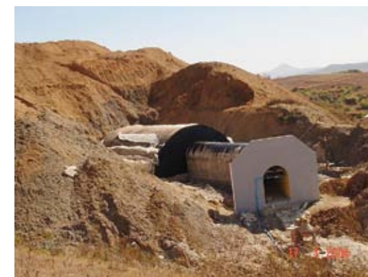
A tortoise shell bunker at neighboring Tigyit was constructed in secret under the supervision of North Korean engineers.
