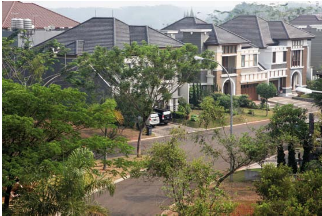
Doxiadis' proposal for three neighborhood plans at varying levels of income used decreasing plot size to accommodate more inhabitants in the low-income areas, however, this design has since been abandoned in favor of a low-density, luxury housing strategy, 2010.
