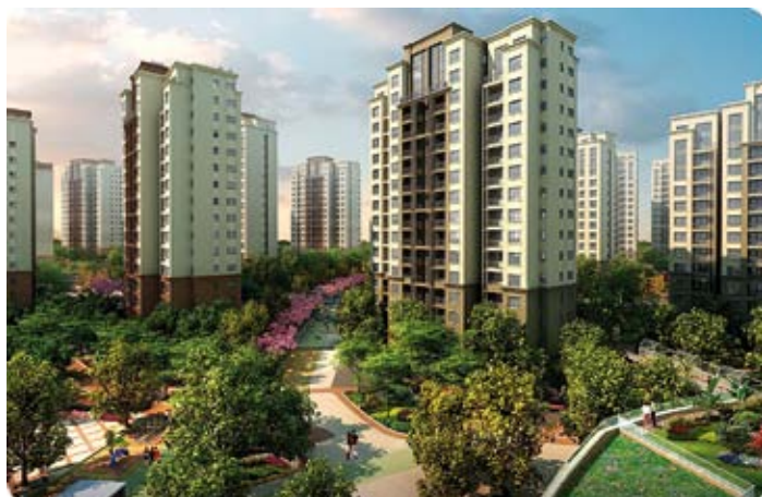
Seasons Park is one of the first residential developments under construction in Tianjin Eco-city. The project is being developed by Keppel Land Corp.
