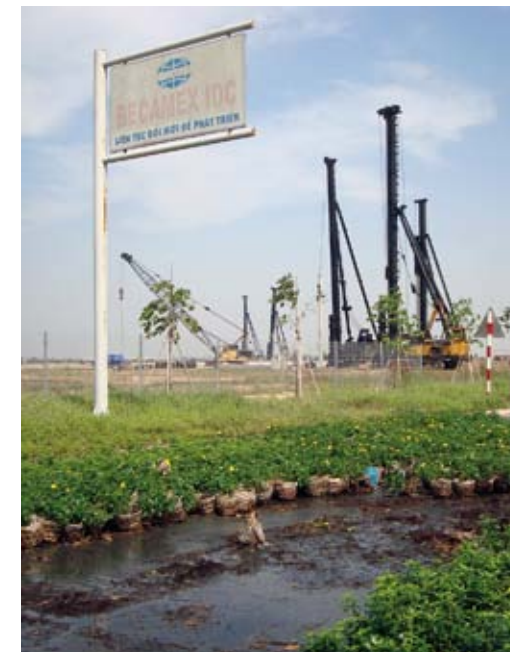
The future administrative area, currently a construction site, 2010.
