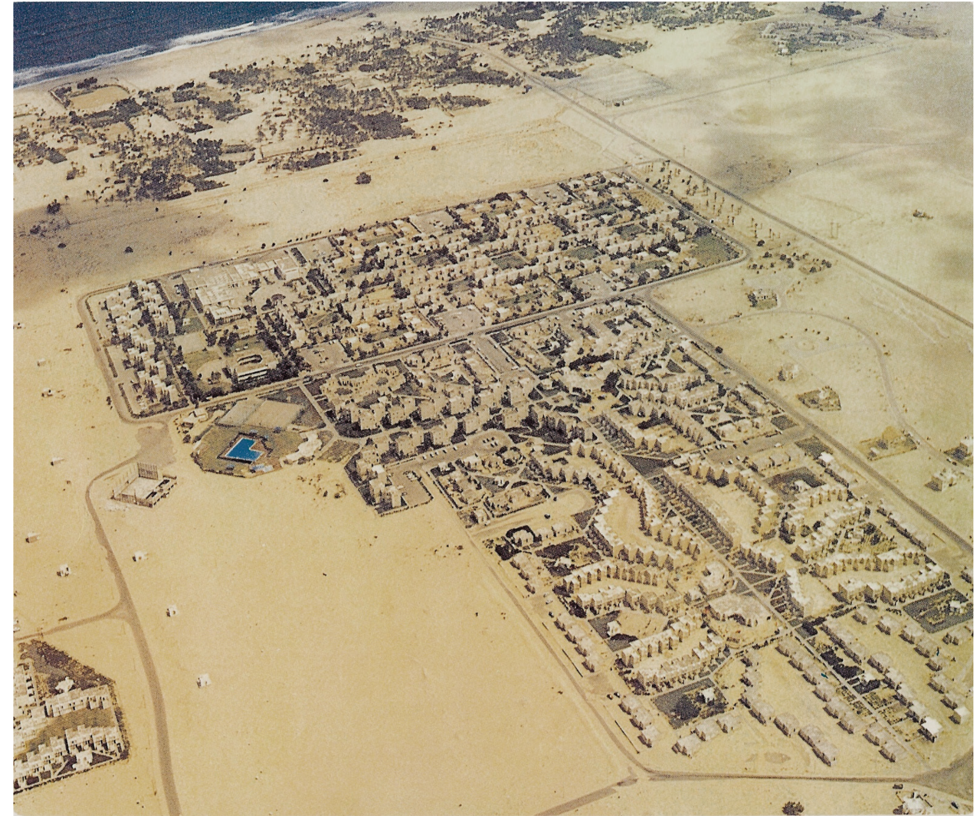
Figure 17: The New Town of Yamit, North-East Sinai. Yamit was built in 1973 and evacuated and destroyed in 1982 as part of the peace agreement between Israel and Egypt. It was the only Israeli New Town physically destroyed.
