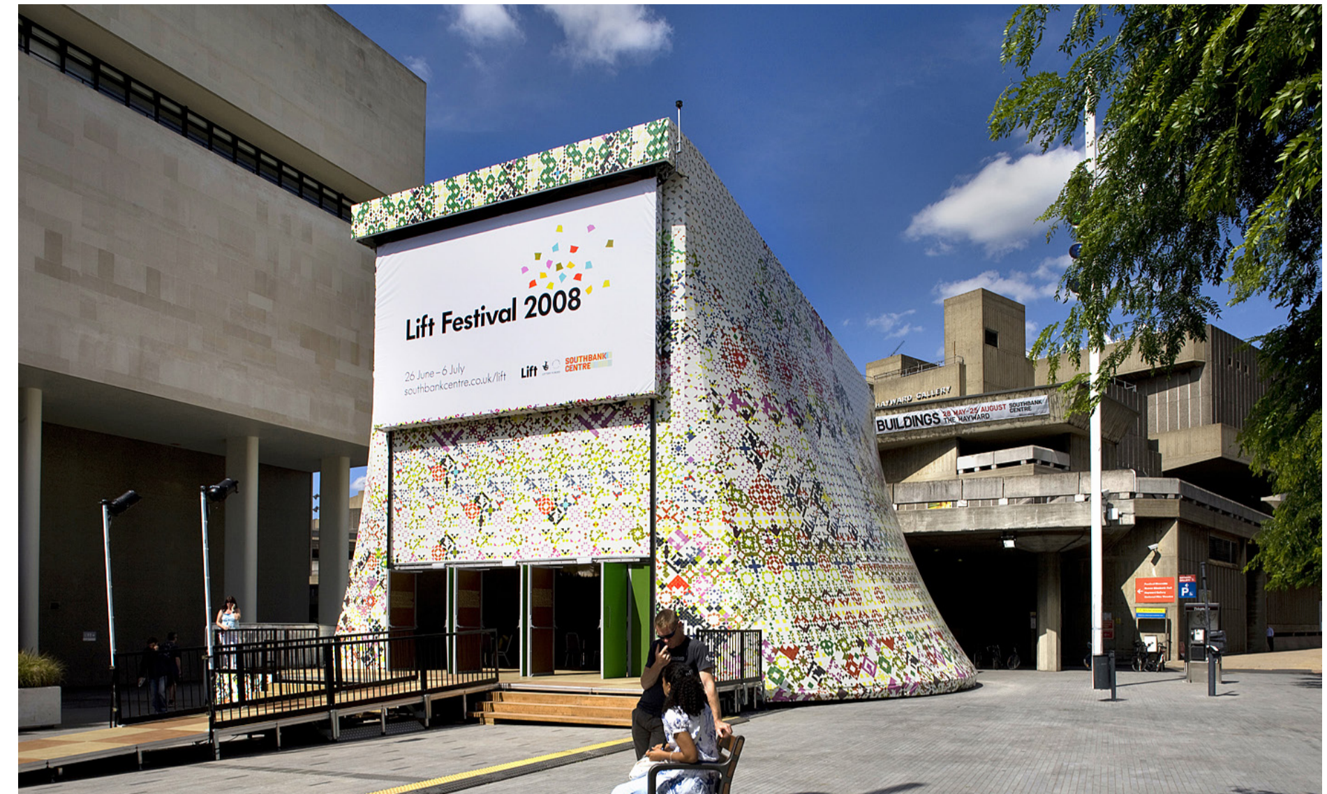
Figure 6: AOC, the Lift, a transportable, demountable meeting and performance space, shown here at the Southbank Centre, 2008. The Lift's very specific shape and external patterned material offers a familiar character and promotes engagement, whilst its kit-of-parts structure and internal deployable roomscape provide endless potential configurations, uses and re-interpretations (Photograph © TBC)
