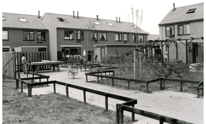
Housing typologies in the in the Vriesland neighbourhood, 1983 Source: municipality of Nissewaard
