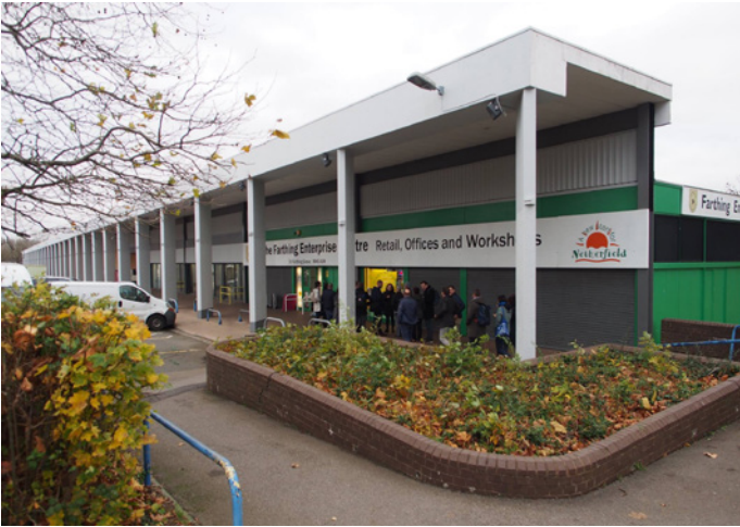
The Netherfield Local Centre, where most shops have closed.
