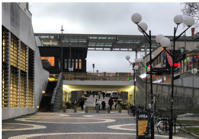
The commercial area Vällingby -Centrum recently renovated. Ph. Will Cousins
