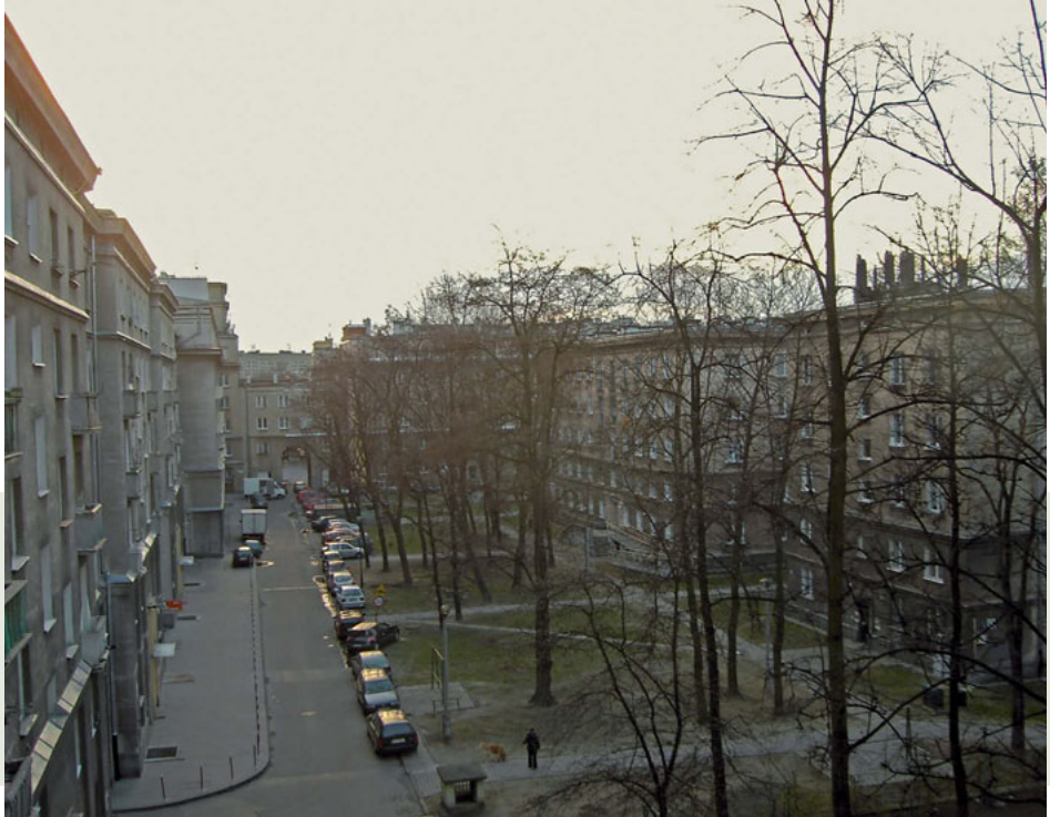
Residential courtyard, Osiedle Centre C-31.
