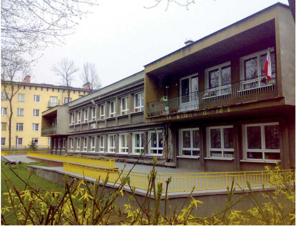
This former school is now converted to housing units.
