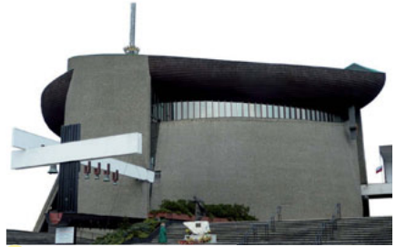
13 The Lord's Ark, the Church of Our Lady Queen of Poland ( Arka Pana kościół Matki Bożej Królowej Polski ) was built between 1967-1977. It was the first Catholic Church in Nowa Huta despite opposition from the communist party and difficulties encountered during construction. The symbolic shape recalls Le Corbusier's Ronchamp chapel, but also refers to Noah's Ark coming to shore on Mount Ararat. The pebble-façade was handmade by volunteers using locally available materials, by architect Wojciech Pietrzyk.
