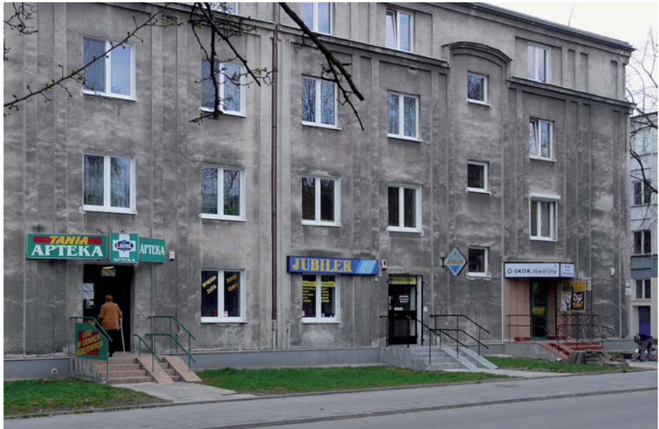
22 An example of ground floor apartments transformed into shops.
