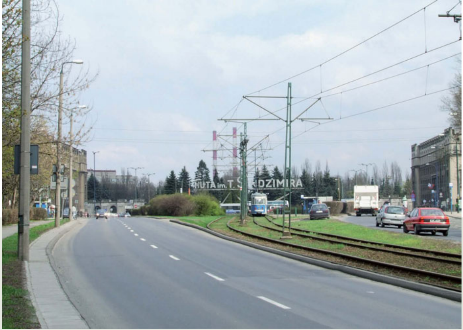
Solidarity Avenue, leading to the Tadeusz Sendzimir Steelworks (HiL).
